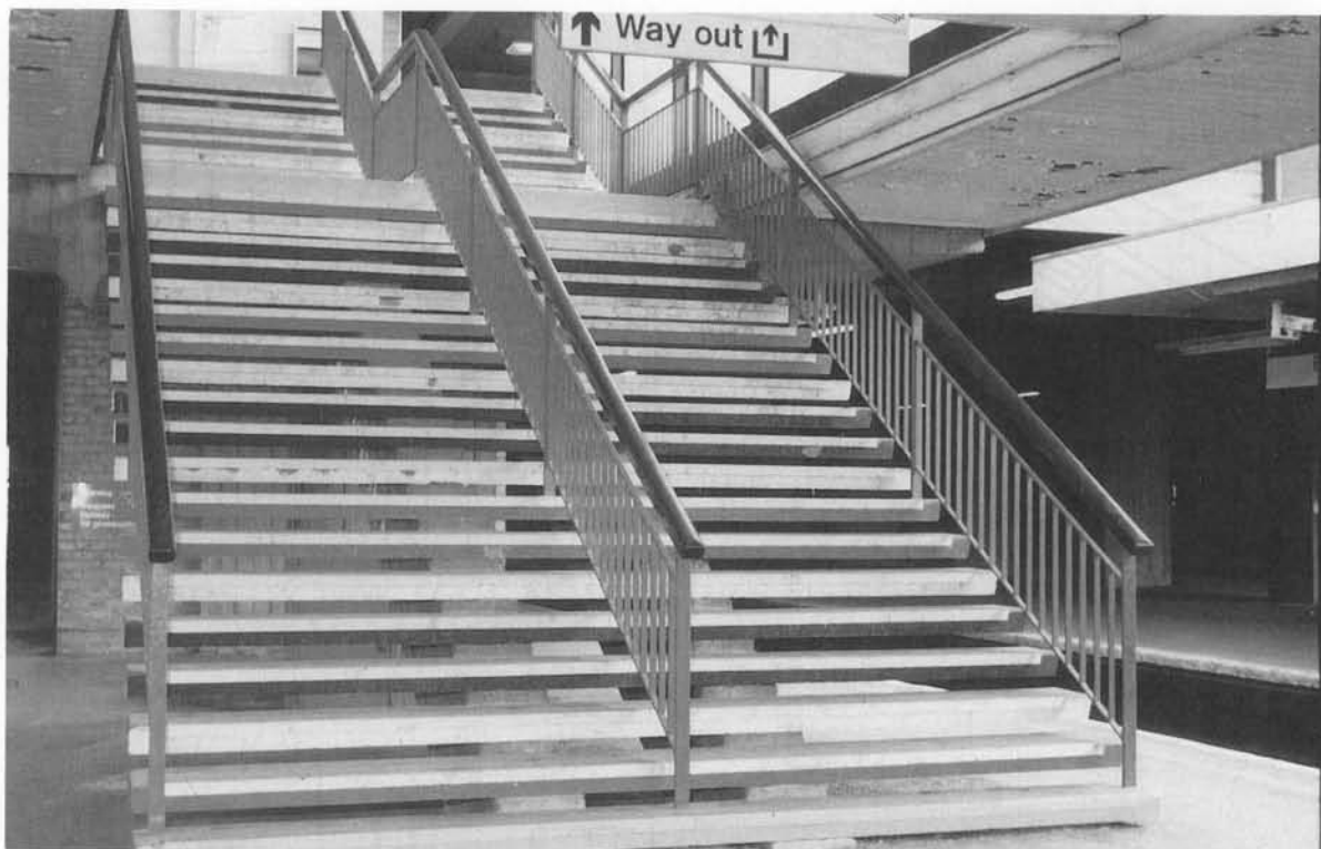
Plate 1.1. Open riser stringer stair straight flight.
