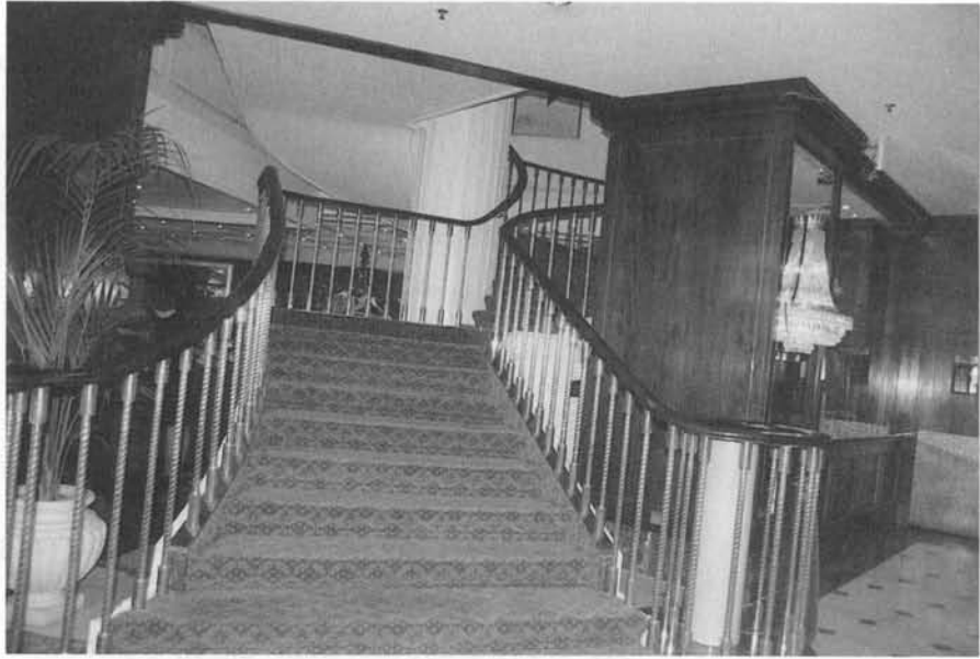
Plate 3.1. Helical staircase in concrete with wood/steel balustrade (with compliments from London Hilton Public Relations Department).
